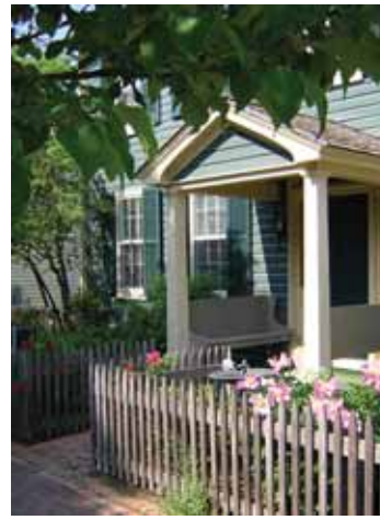
Wood picket fence at front sidewalk
