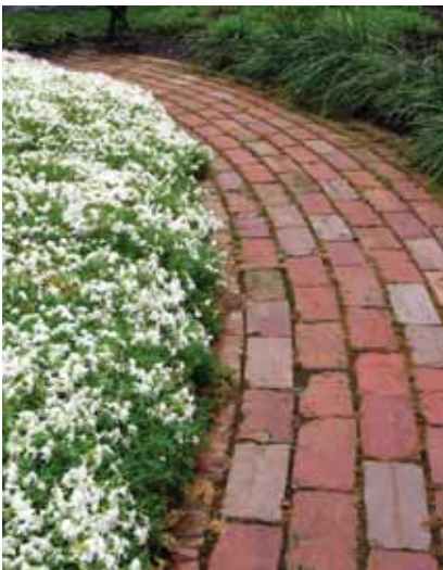
Pervious paving to aid in percolation of runoff water
