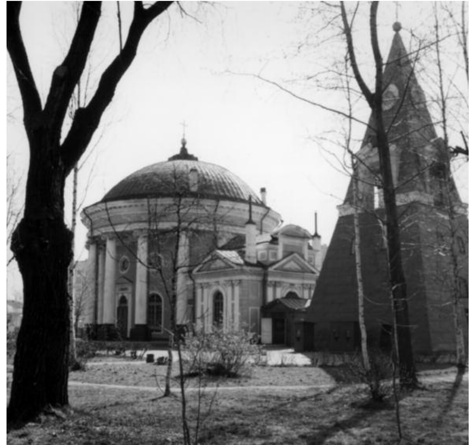
FIGURE 8: Church of the Trinity, Viazemskii Estate, Aleksandrovskoe (southeast outskirts of St. Petersburg). Nikolai Lvov, architect.
