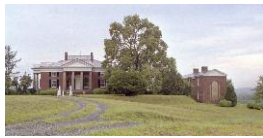
Figure 3. Front facade, with view after wing of the right. (Reverend)
